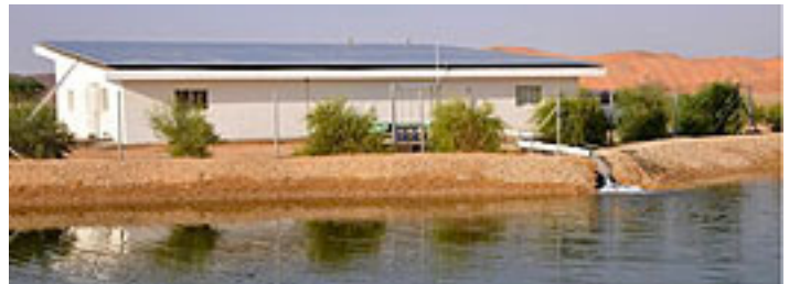
A Solar-powered BWRO Plant
